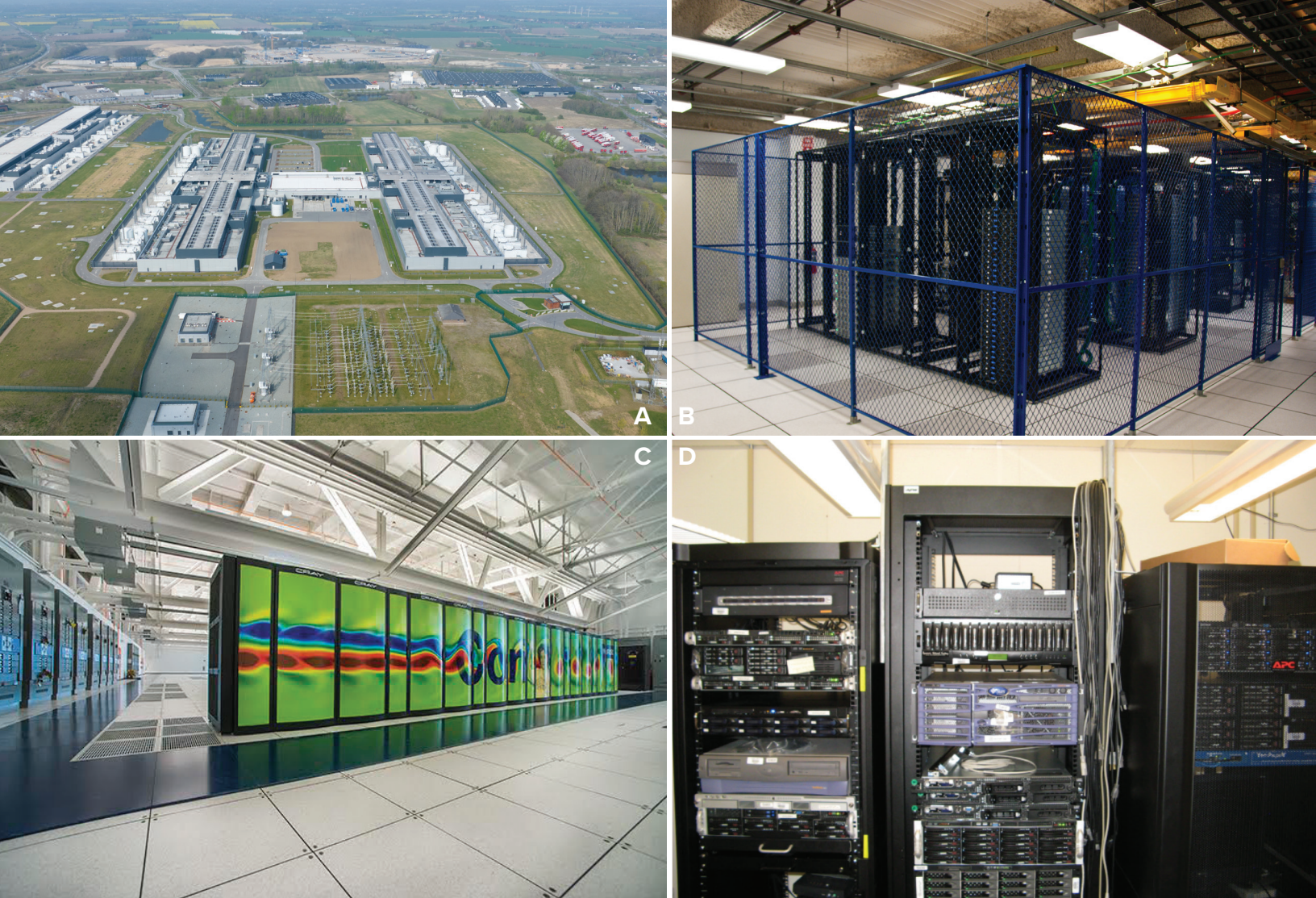
Figure 1-1. The many shapes and sizes of data centers: (a) Meta's hyperscale data center campus in Odense, Denmark, which contains more than 200,000 m 2 of floor area 10 ; (b) an example of a tenant-leased space in a co-location data center with secured access 11 ; (c) a high-performance computing (HPC) data center occupying around 13,000 m 2 12,13 ; and (d) a small data center room in an office building, occupying less than 100 m 14 .
