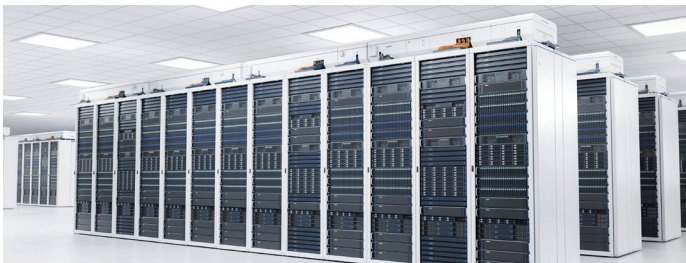
Figure 1-3. A typical data center information technology (IT) equipment layout with individual IT racks arranged in rows. In this depiction, each row contains 13 racks.
